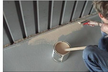
**Start Painting:** After material is thoroughly mixed, Start Painting in the corner furthest away from the exit of the room. Use a brush to cut in along the walls, use a roller to roll material on floor surfaces away from the wall.
