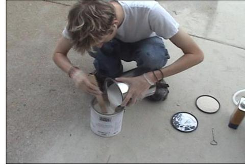
**BASECOAT MIXING INSTRUCTIONS:** Slowly add Basecoat Part B to Basecoat Part A in a 1:1 ratio. (Entire half-gallon to half-gallon). Stir thoroughly and scrape sides of can to ensure thorough blending. Allow the mixed material to stand 45 minutes at temperatures below 70°F (21°C) before use. Above 70°F (21°C) allow 30 minutes induction time. Always restir before use. Mixed material is usable for six to eight hours. Do not thin with solvents use water if thinning is
