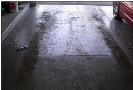
**Previously Painted Surfaces:** The waterborne components of this product generally allow use over most old coatings. Old coatings should be tested for lifting. If they lift, remove them. Wash to remove contaminants. Rinse thoroughly with water and allow to dry. Dull glossy areas by light sanding. Remove sanding dust. Remove loose paint. If no lifting, lightly sand the surface and clean with TSP (*Trisodium phosphate*) or substitute.
